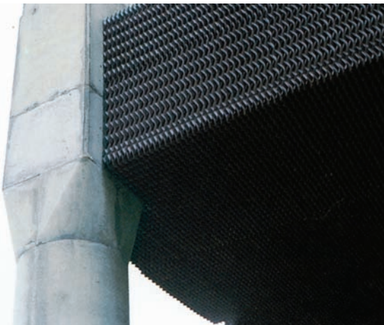
Unobstructed Marley counterflow fill installation
