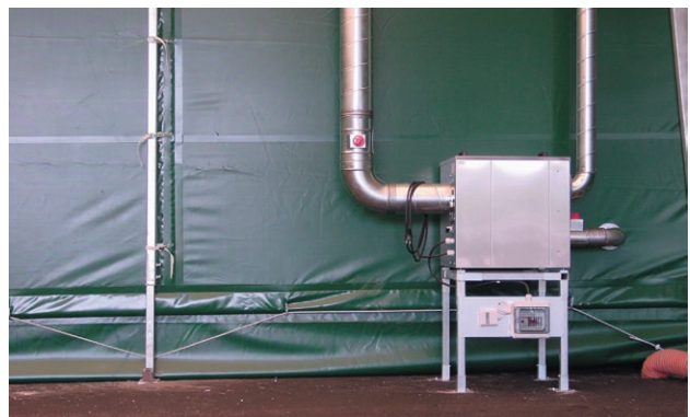
DST dehumidifier Recusorb DR-40 installed in a plastic storage tent
