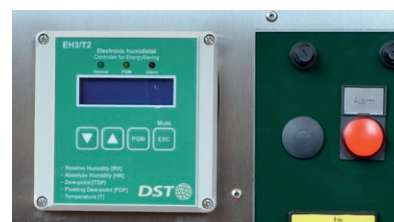
EH3 T2 mounted in a R-61R dehumidifier
