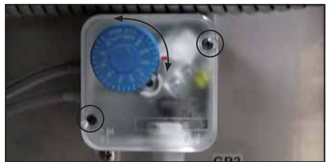
FIGURE 8: E.g. Electronic filter guard with warnings lights combined with pressure gauges
