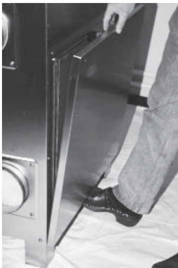
Removal of door
