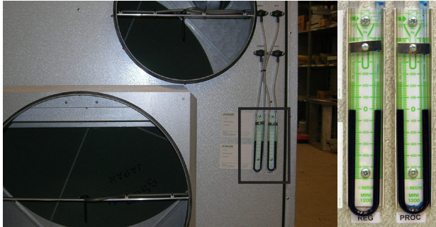
FIGURE 11: Differential U-tube manometers
